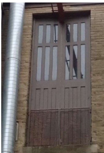
Existing First Floor Doors
